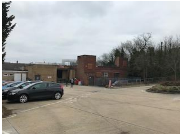
Rear of the property/service yard onto Town Hall Car Park
